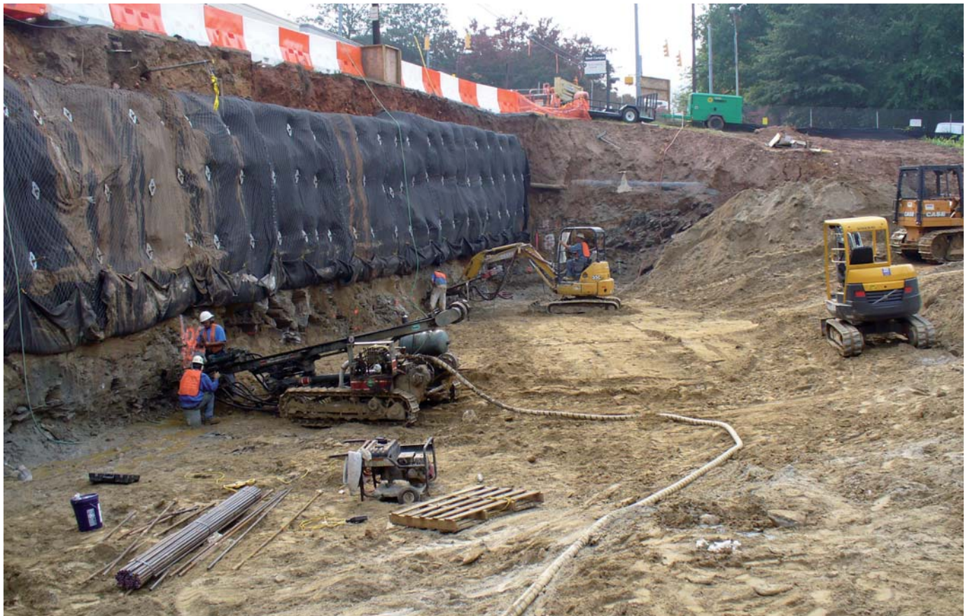
Figure 14: Fabricating the temporary shoring wall
