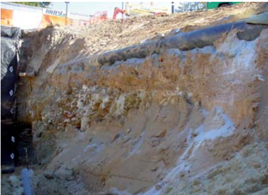
Figure 10: Water service line embedded in the slope.
