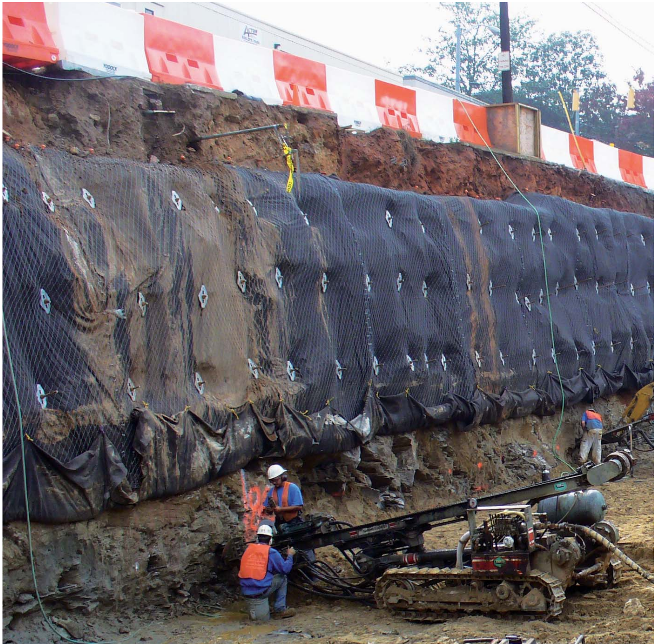
Soil nailing and anchoring in a temporary shoring application
