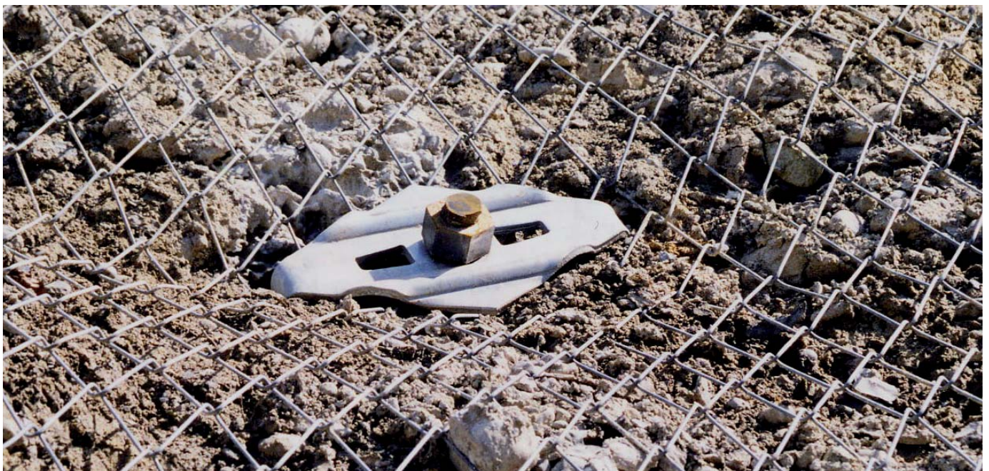
Figure 9: Pre-tensioning
