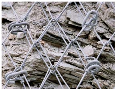
Figure 8: Mesh connection with compression claws
